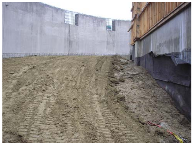
Completed ramp wall
