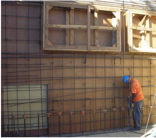
Preparing the wall of the Bicycle Room and Emergency Generator Room
