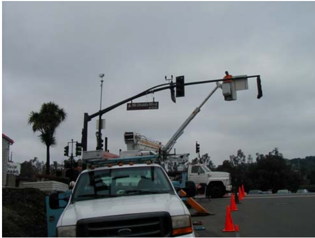
New traffic signals at Mount Diablo Boulevard and First Street for new traffic movements that are required for the LLLC
