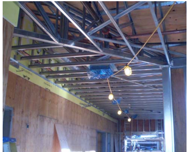
Completed truss work in the Community Hall's Gallery
