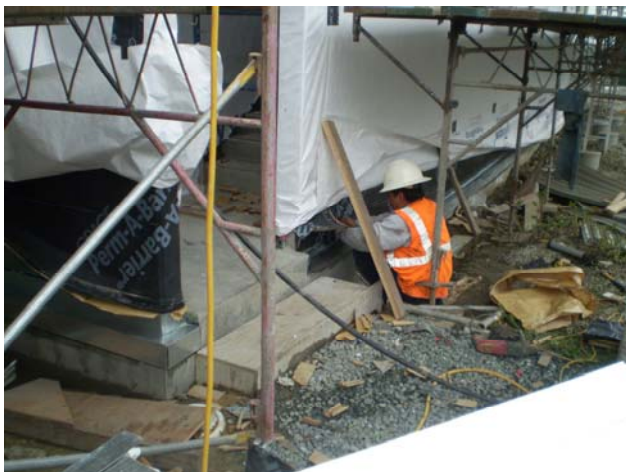
Adding flashing around exterior ground edge
