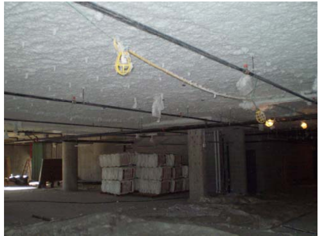
Blown insulation in the ceiling of the First Level garage
