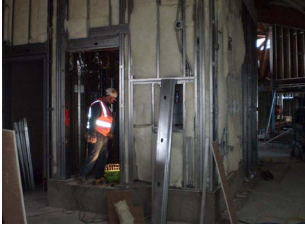
Insulation being added around the Copy Room
