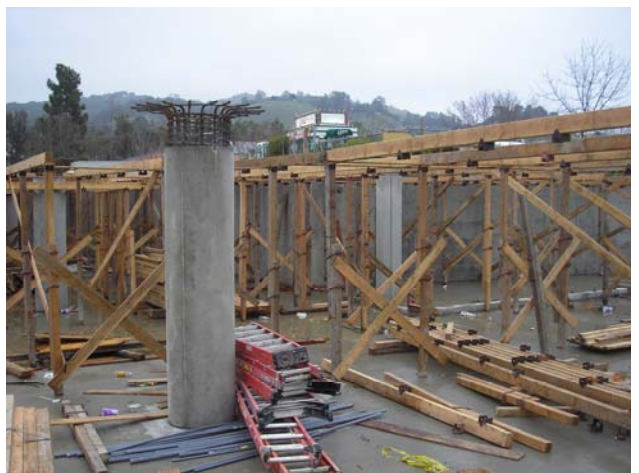
Formwork for Second Level
