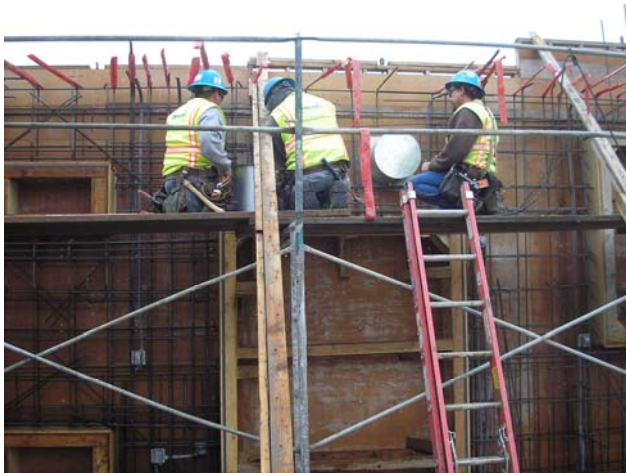
Installing sheet metal in walls of First Level parking area
