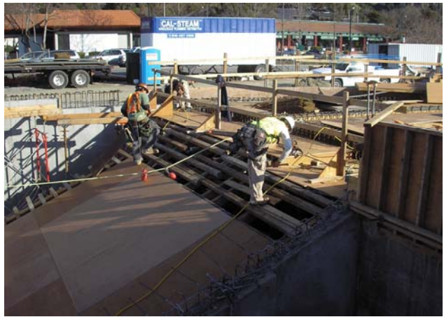
Preparing the forms for the Plaza Staircase
