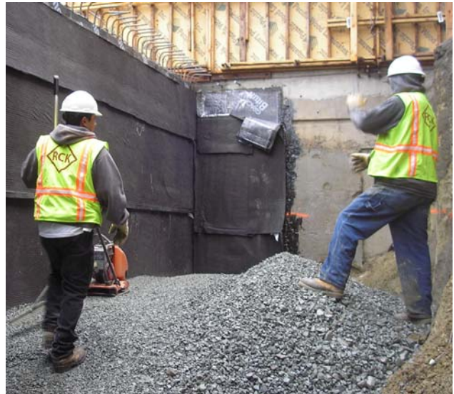
#4 – Gravel is spread by hand.
