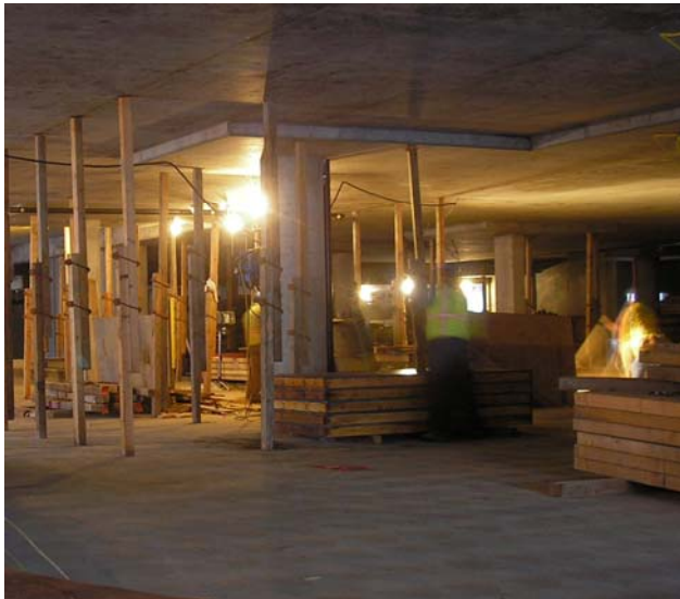
Removing forms in the First Level parking garage
