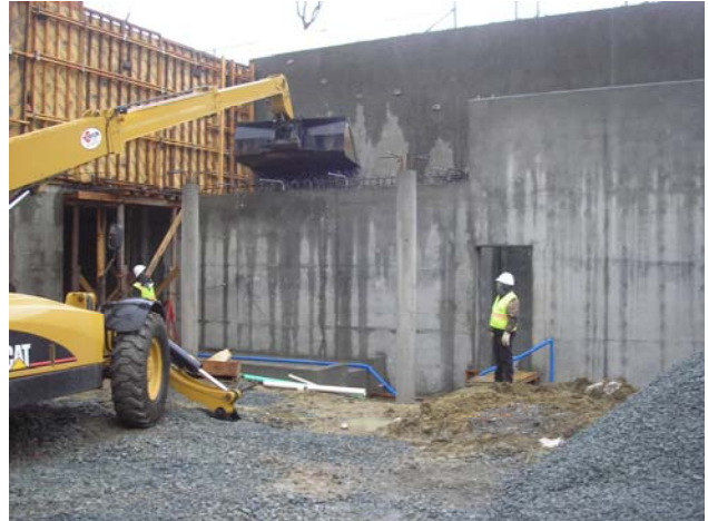
#2 – Gravel is lifted over the wall.
