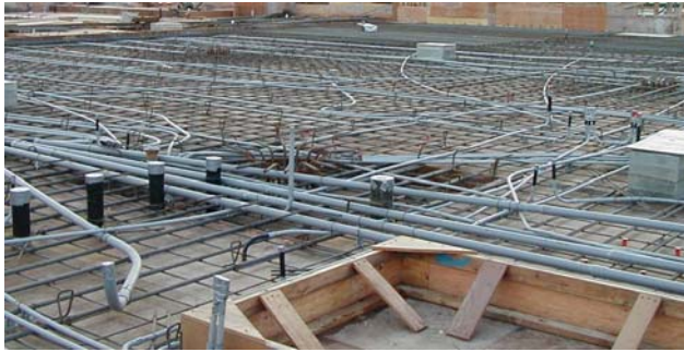
Rebar and conduit on the Second Level
