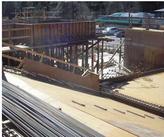
Looking down the Plaza Staircase into the Reading Court below
