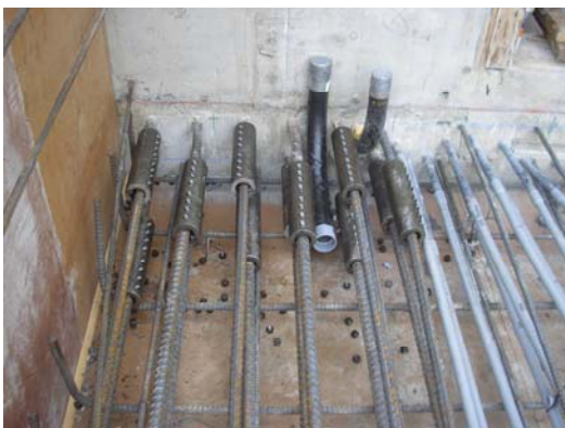
Rebar tie-ins to a wall
