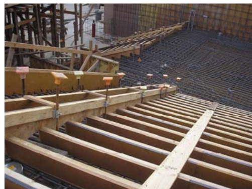
Step forms completed
