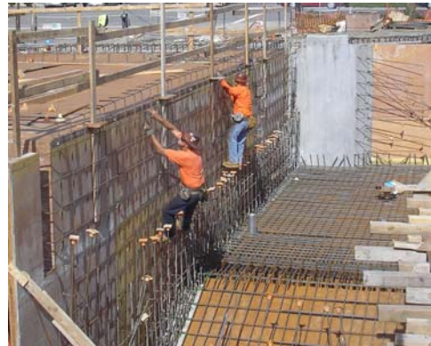
Wall of Community Hall next to the Plaza Stairs
