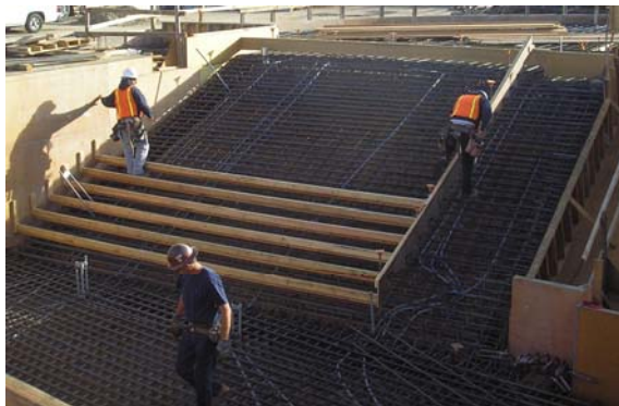
Forming the steps for the Plaza Stairs
