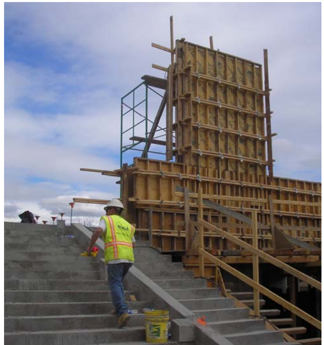
Wall for elevator at the Main Level Lobby
