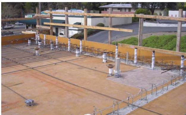
Plumbing connections for Community Hall restrooms
