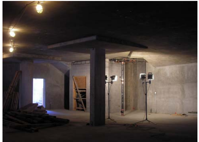
Elevator to the Main Level Lobby at the First Level parking area
