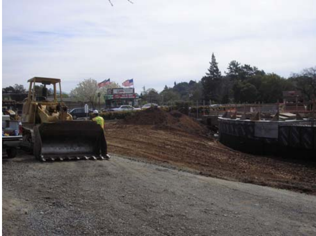
Backfilling and grading on the north side
