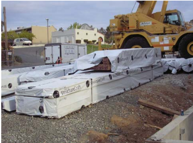
StructureCraft components arrive on-site
