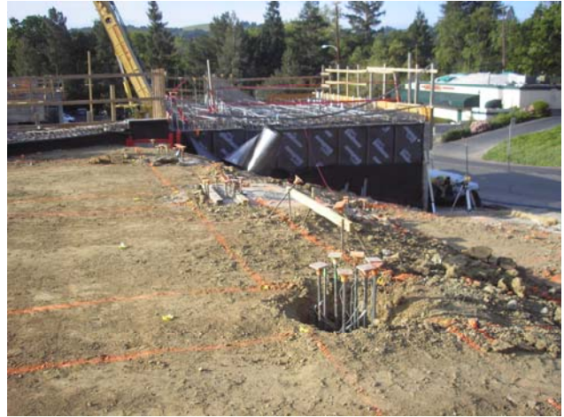
Pilings for the Community Hall
