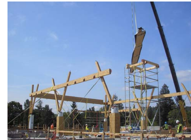
Installation of heavy timber system in the main library space
