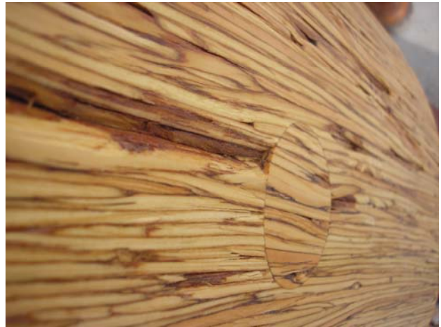
Details of truss lamination
