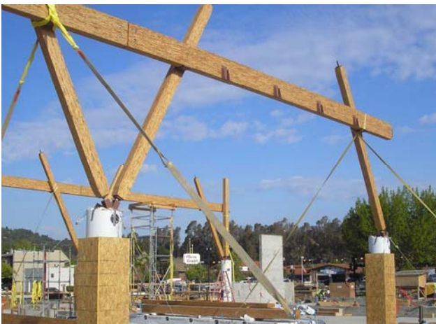
Installation of heavy timber system in the main library space
