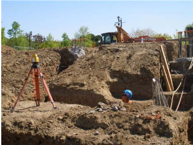
Excavation for Community Hall foundation
