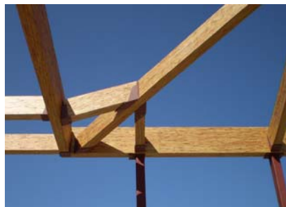
Forming of the truss joints prior to raising
