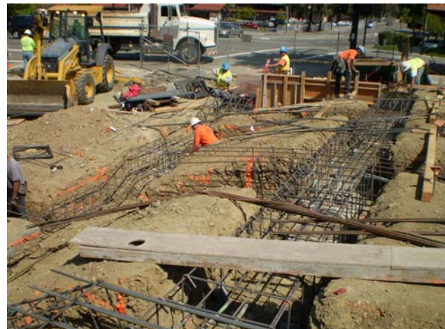
Forming rebar for Community Hall foundation
