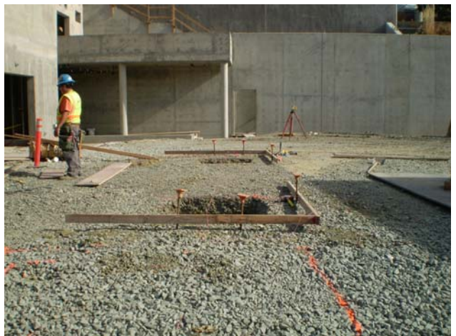
Pier excavation for drive-thru book drop canopy
