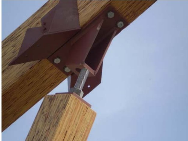
Truss connection
