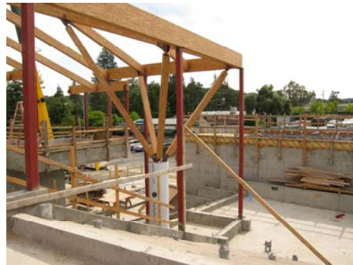
From the top of the Main Staircase
