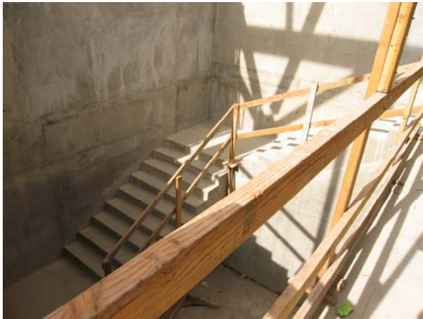
Interior staircase to the parking garage
