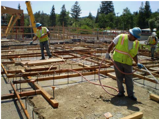
Community Hall foundation
