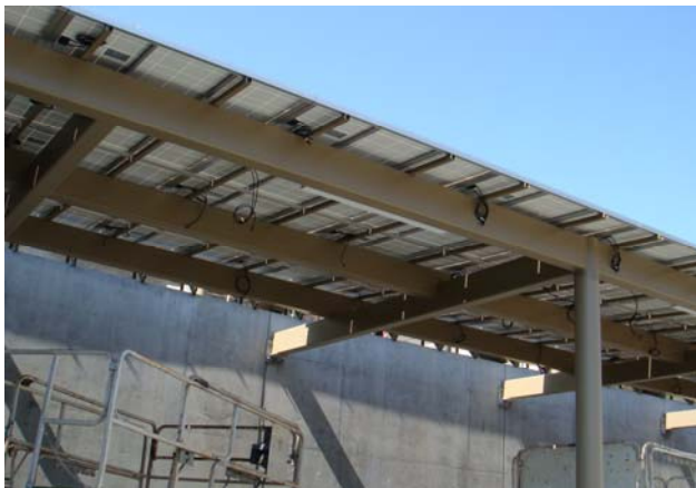
Solar panels in parking lot
