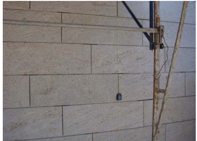
Plumb line for installing granite
