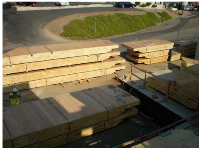
Staged roof panels
