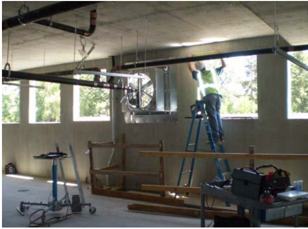
Installation of parking garage exhaust fans
