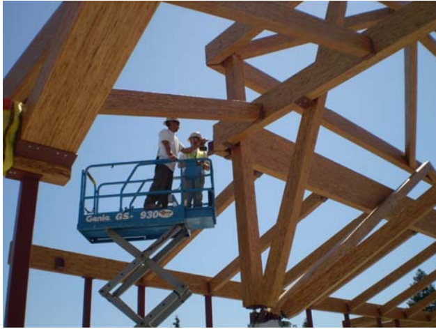
Completing connections in truss system
