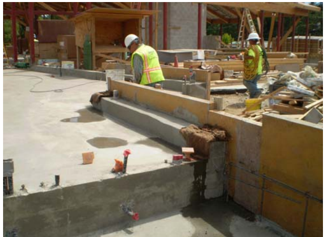
Wall foundations in Staff Wing
