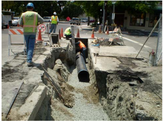
Storm drain in Golden Gate Way
