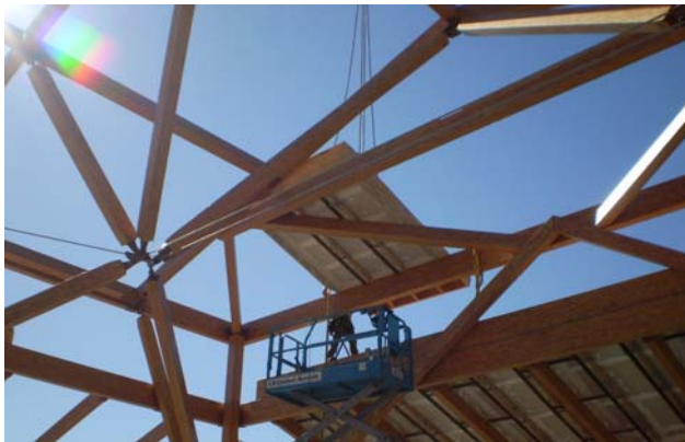
Installation of roof panel
