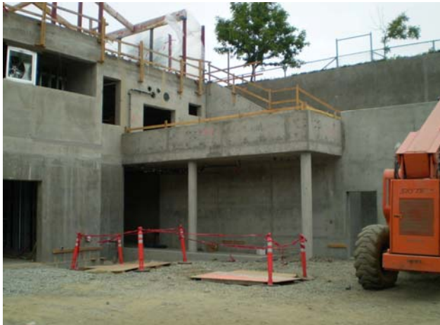
Looking northwest from the parking lot
