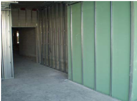
Interior walls in the Arts & Science Discovery Center
