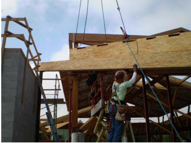
Installation of a roof panel
