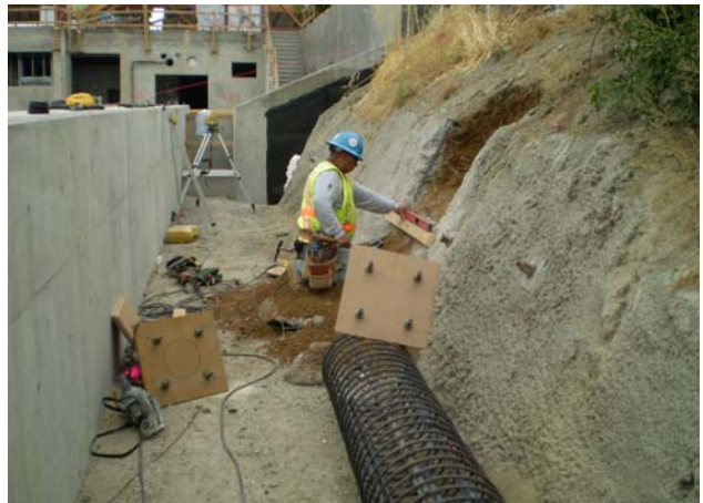
Preparing the pile foundations for the second tier of the solar panels
