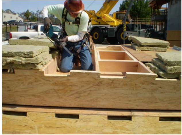
Insulation within the roof panel
