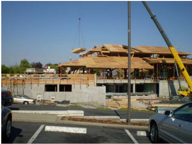
Installation of a roof panel
