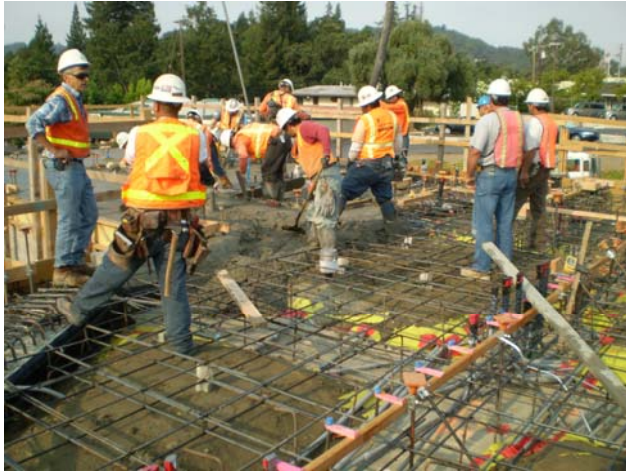
Pouring the Community Hall sub-floor
