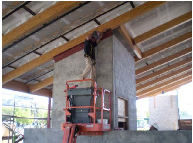
Securing the roof to the Main Elevator wall
