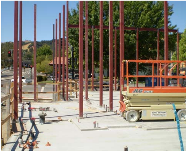
Steel framing for the Community Hall walls
