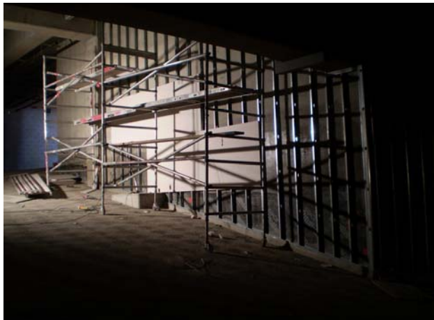
Installing wall panels on the Parking Garage ramp
