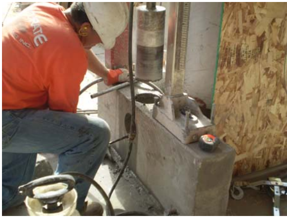
Concrete coring
