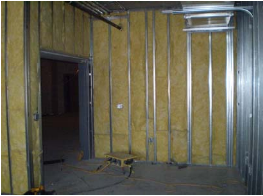
Insulation in wall panels
