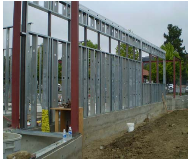
East wall of the Staff Wing with clerestory windows
