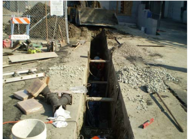
Installation of the main sanitary sewer line
