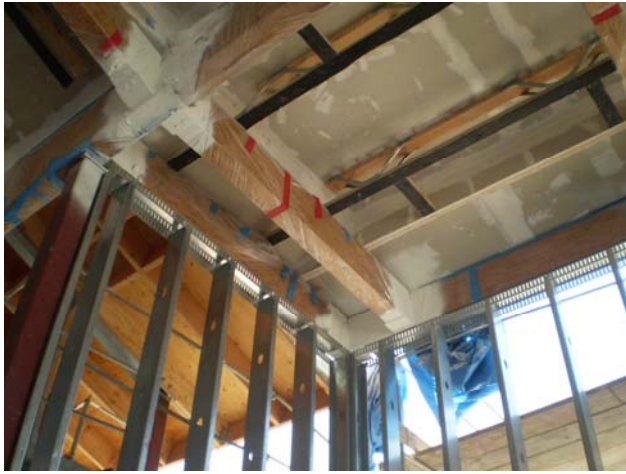
Joining the roof structure with interior walls
