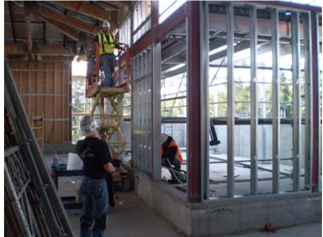
Framing the west wall of the Homework Center
