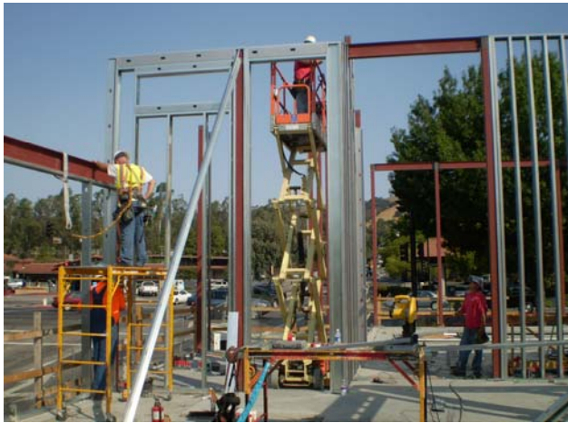
Framing of the northwest corner of the Community Hall
