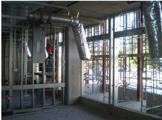
Ductwork being installed in the Arts & Science Discovery Center
