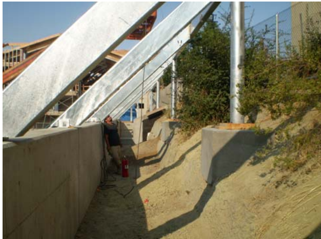
Supports for the upper tier of the solar panels
