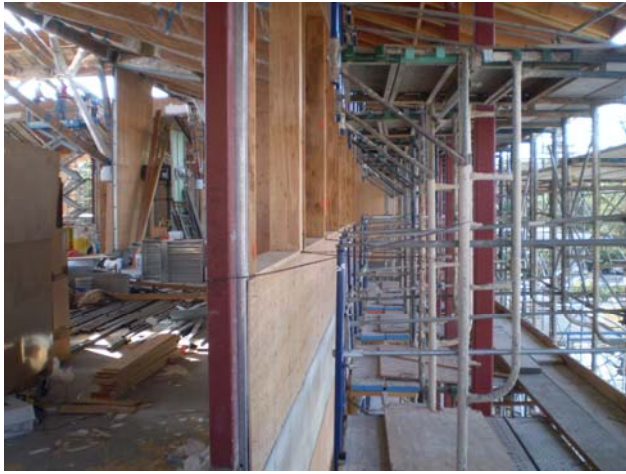
Framing of west wall of the Technology Lab
