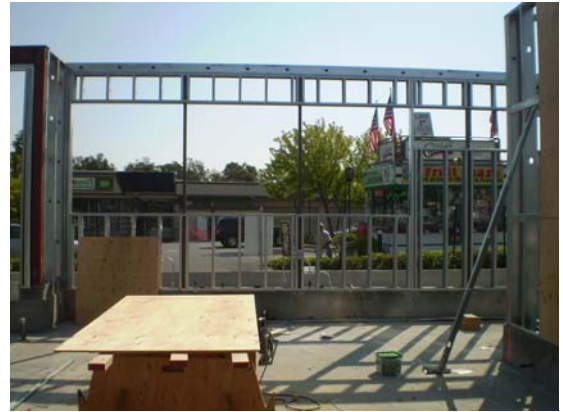
Viewing through the east windows of the Staff Workroom
