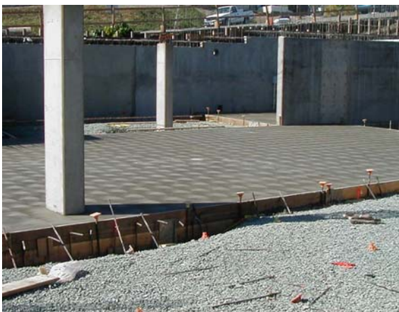
Final floor finish of the parking area in the Basement
