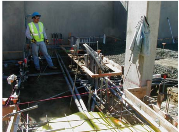
Installation of conduits in the Main Electrical Room
