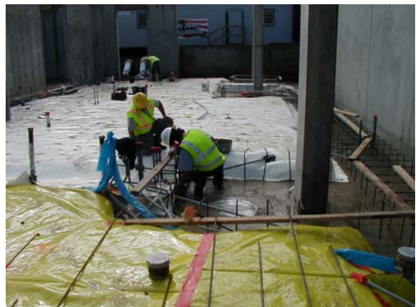
Installation of waterproofing in the Friends Book Room
