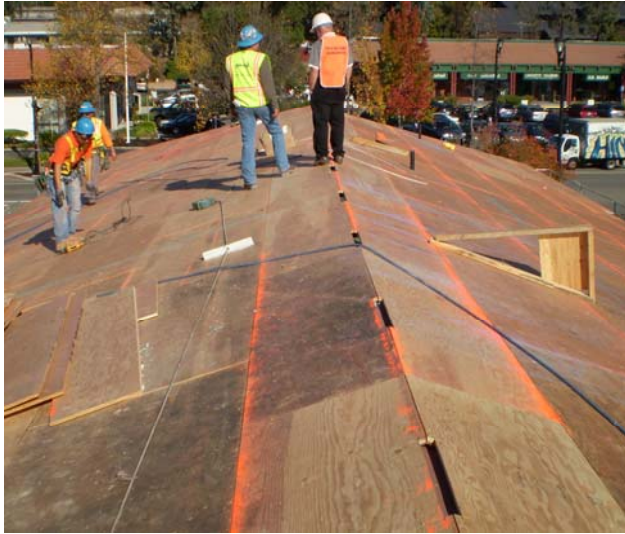
Roof of the Staff Wing before the weatherproofing was installed
