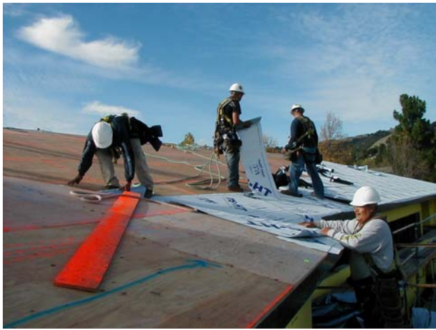
Weatherproofing the roof
