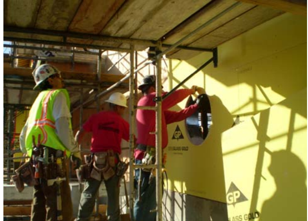
Cutting the wall board around one of the Big Dipper windows
