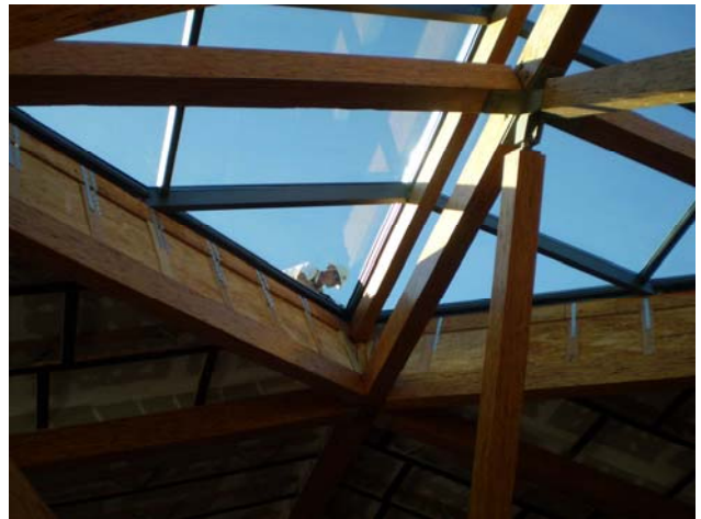
Skylight over the Children's Area
