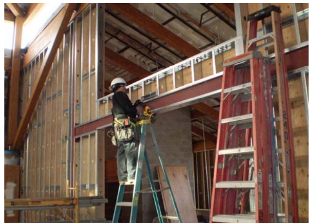
Installation of the EXIT sign box in the main Library space
