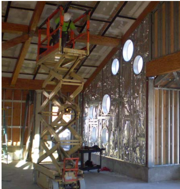
Interior insulation around the Big Dipper windows in the Children's Area
